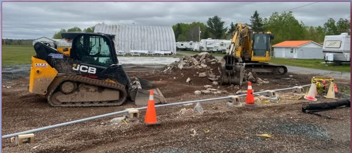
Work underway on the reconstruction of buildings lost to last year's fire. PHOTO by Leonard Lowe
