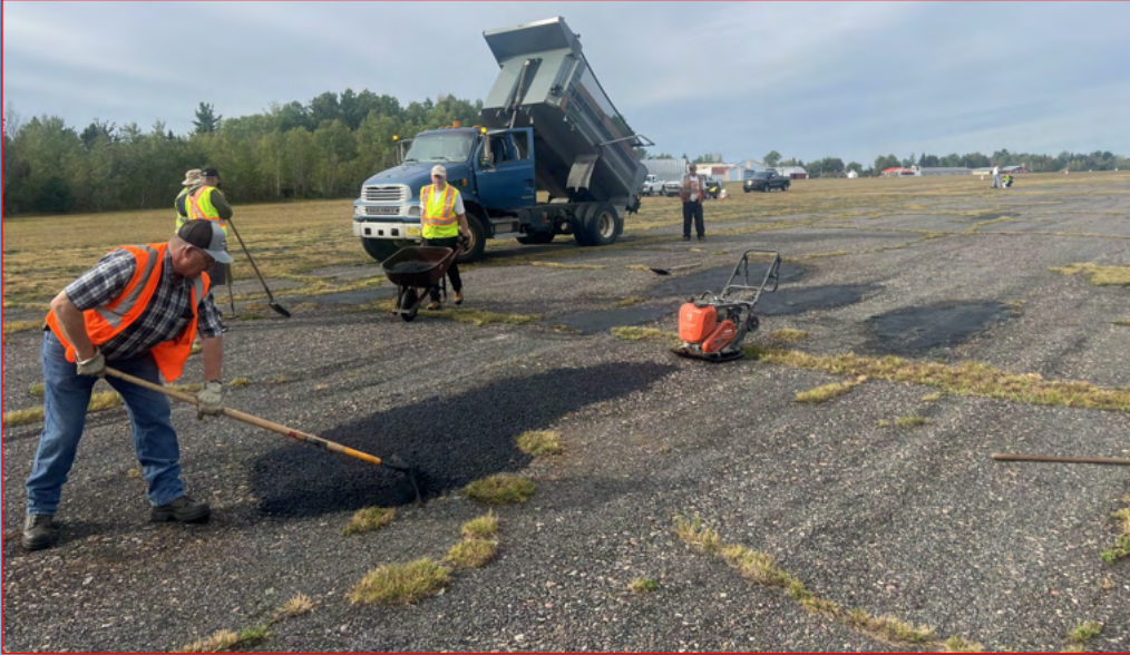
SSAA members work on runway restoration. PHOTO by Jim Ward
